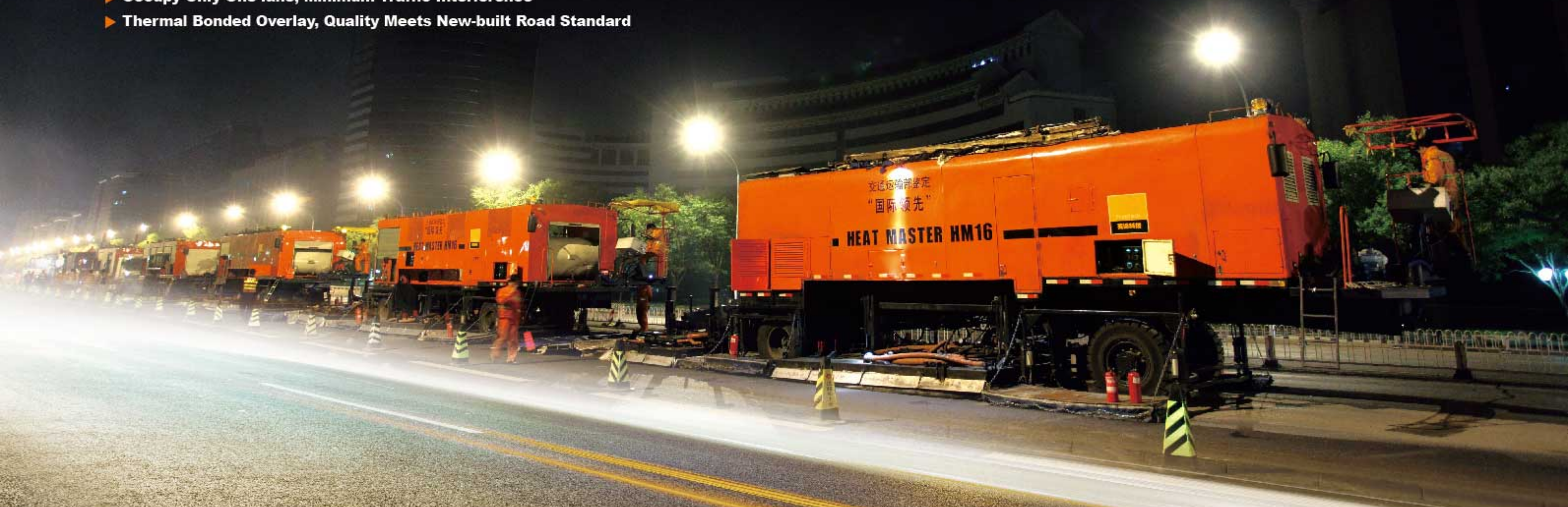
Recycling Project of Chang'an Avenue, Beijing, China ▲
